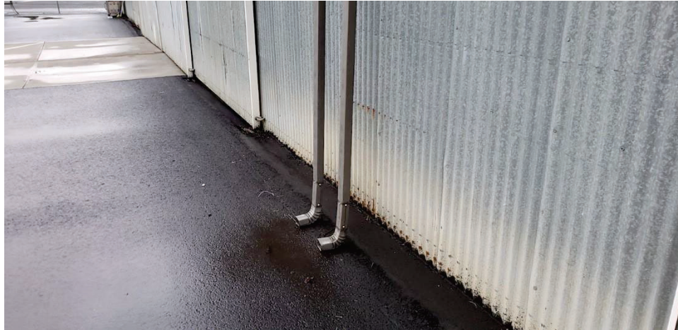
Pavement and Gutters Installed; Photo: Jury Member
