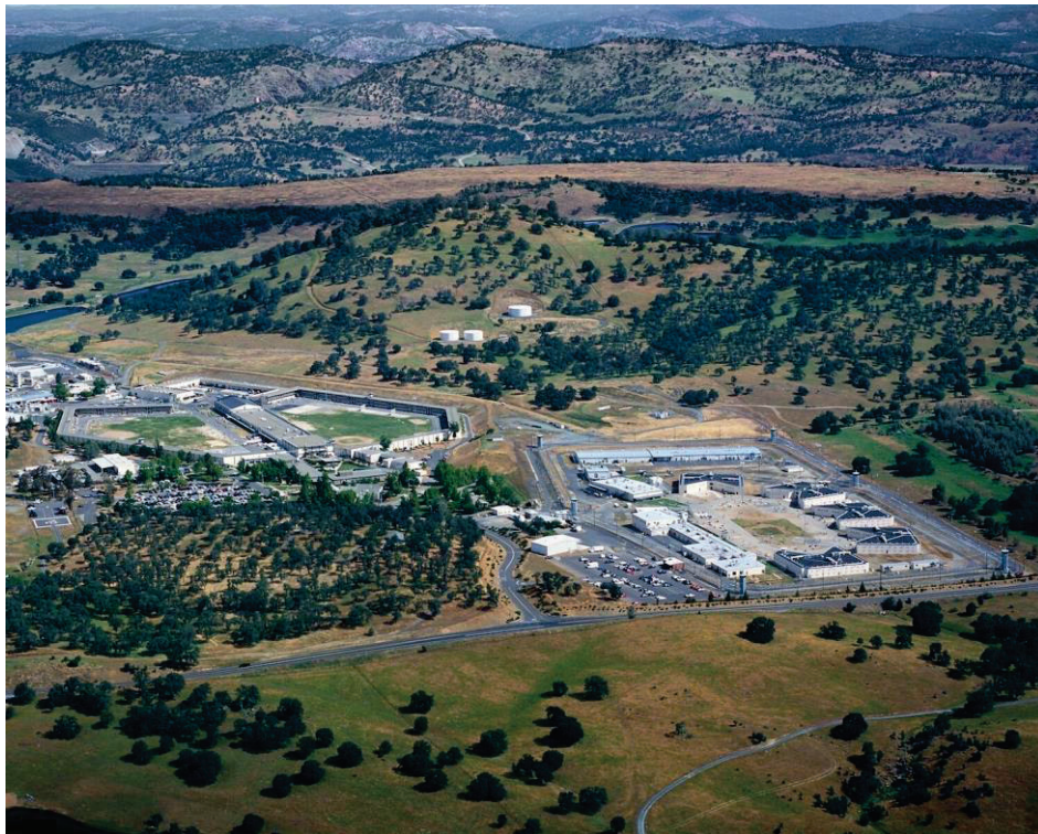
Sierra Conservation Center Photo provided by Department of Corrections and Rehabilitation
